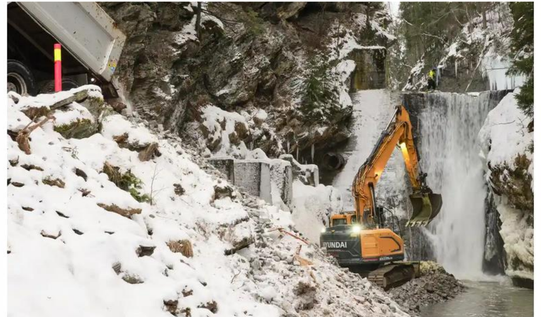
📷 Campaigners say removing the seven-metre dam, in Fåvang, Norway, which has not been used in
